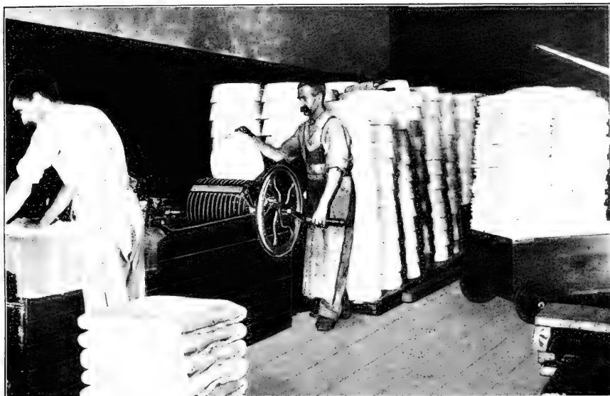
GRINDING AND PRESSING CRUDE SPERMACEI FOR REMOVAL OF TAUT-PRESSED OIL.
